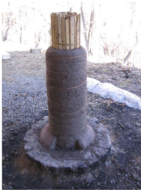
Figure 4.2.: Fully constructed bloomery [36].
