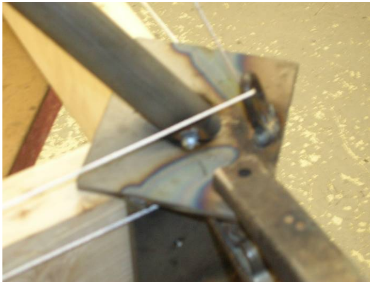
Figure 26: Close Up of Corner Bracket with Supporting Pole Tacked in Place
