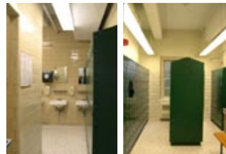
Existing locker rooms
